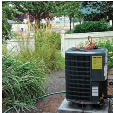
An air-source heat pump compressor located outside the house can distribute hot and cold air through your existing duct system. Photograph by Peter Stevens
