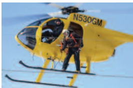
Installing bird flight diverters
