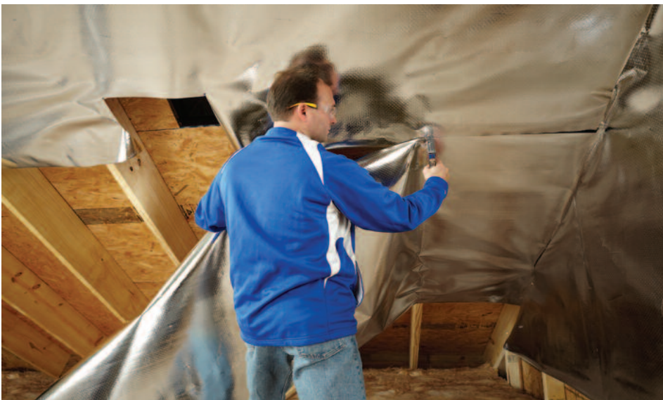
Foil is placed under the framing supporting the roof, reflecting unwanted radiant heat upward and out of the home. Photograph provided by Reflective Insulation Manufacturers Association International
