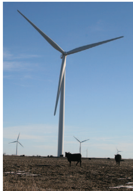
Wind is used to produce electricity by converting the kinetic energy of air in motion into electricity. The wind rotates the rotor blades, which convert kinetic energy into rotational energy. This rotational energy is transferred by a shaft to the generator, producing electrical energy. Photograph by Wayne Price
